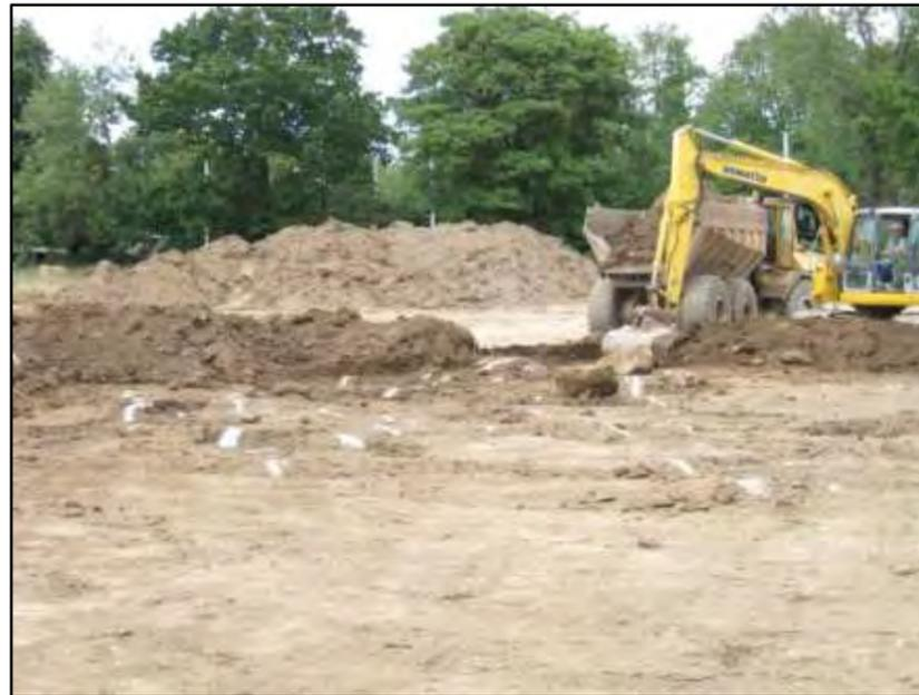
Plate 8: View (from southeast) of topsoil clearance at Priorsland temporary Park & Ride. Note concentration of granite boulders.
