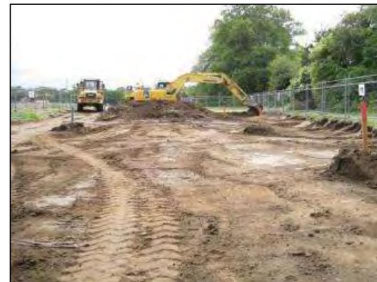
Plate 3: View (from west) of topsoil clearance along access road to Priorsland temporary Park & Ride.
